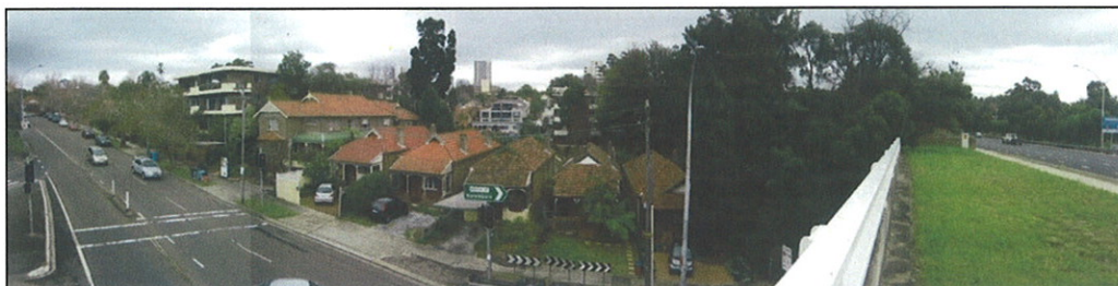
Photo 1: View of the site
